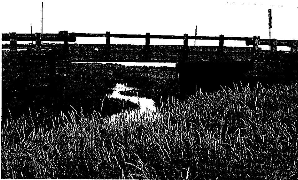
Figure 3.4. Bridge 1 (looking east).
