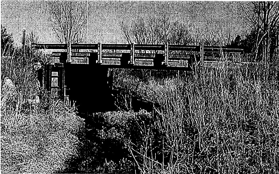
Figure 3.12. Bridge 2 (looking north).
